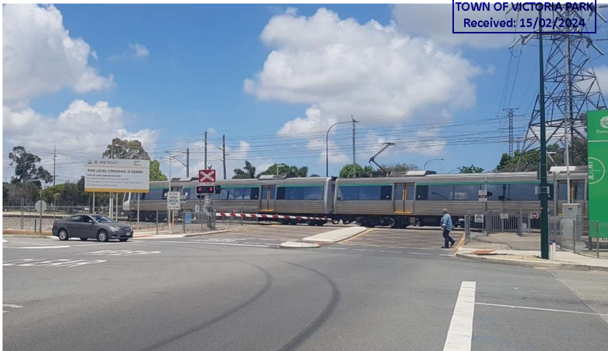
Photo 10: Keep clear markings allow some turns to / from the side road during level crossing closures.
