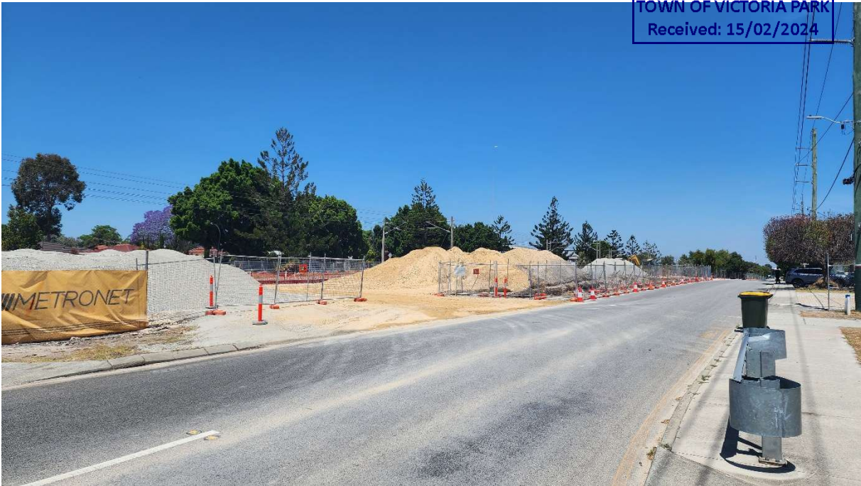
Photo 6: This area is earmarked for a relocated bus interchange.
